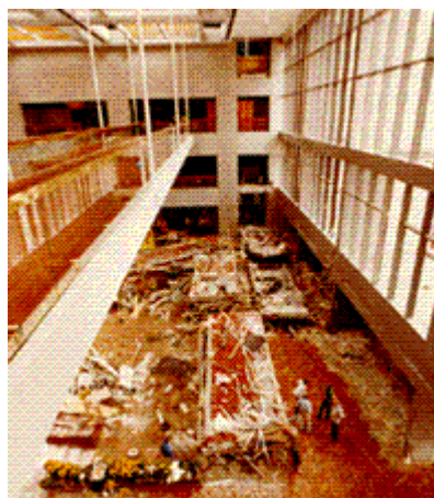
Figure 3.2b : Hyatt Regency Walkway, après.
